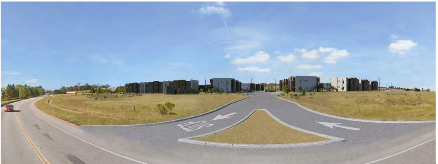
From R-DEIR fig. 4.1-18a: “View from Glenn Coolidge Drive with Project (6 Months Growth)”
